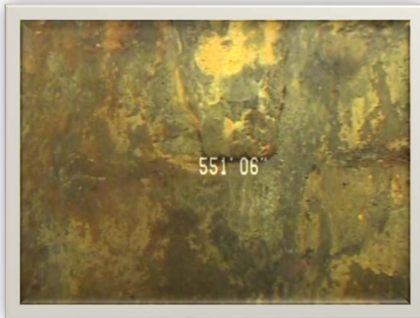
Videograph A2: View of one of the sawteeth bottom of upper casing liner. Note the plugged perforation to the right of the sawtooth.
