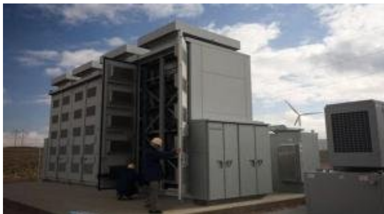
Figure 3 Lead-Acid Battery Storage
