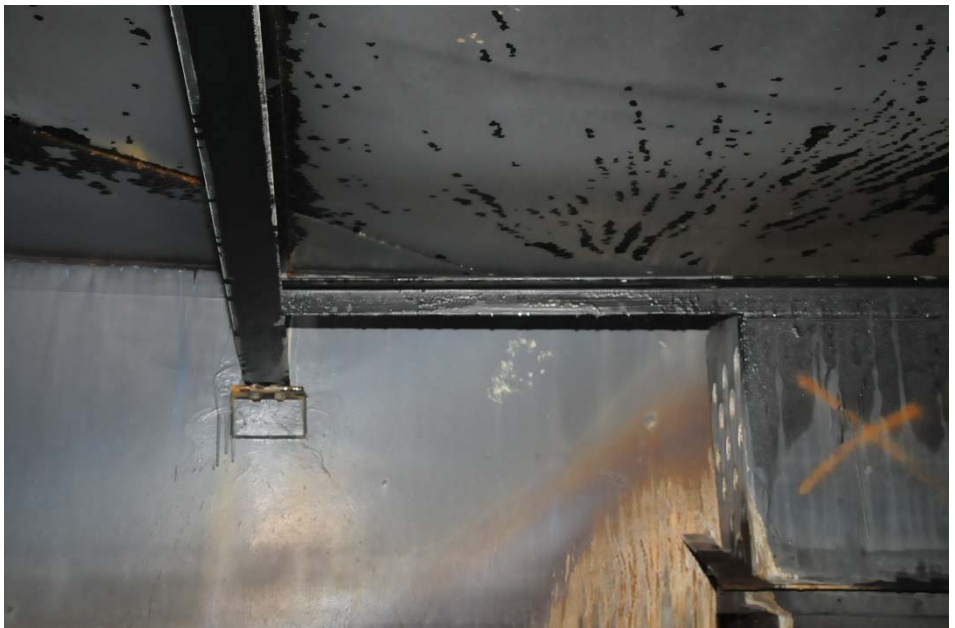
I-28 View of an angle supporting the weir box between rafters, illustrating generally good condition of the coating system.
