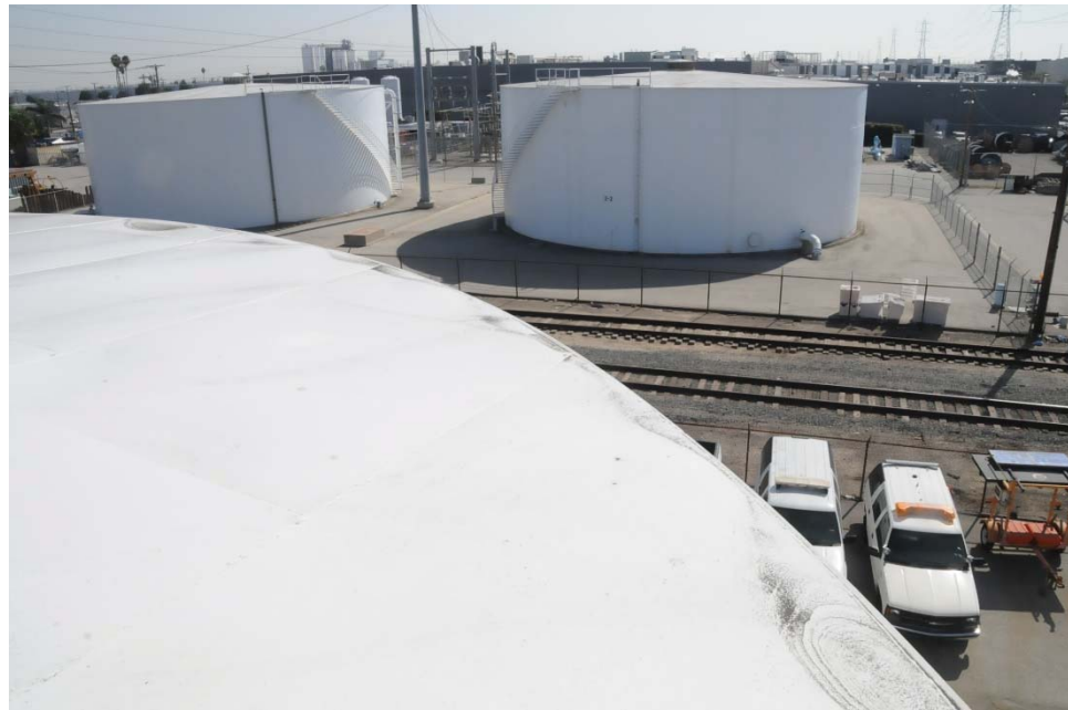
E-15 View of the perimeter of the roof, illustrating staining and otherwise good condition of the paint system.
