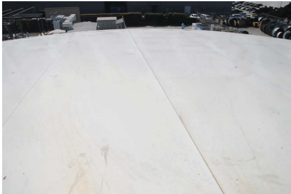
E-8 View of a portion of the roof, illustrating generally good condition of the paint system.
