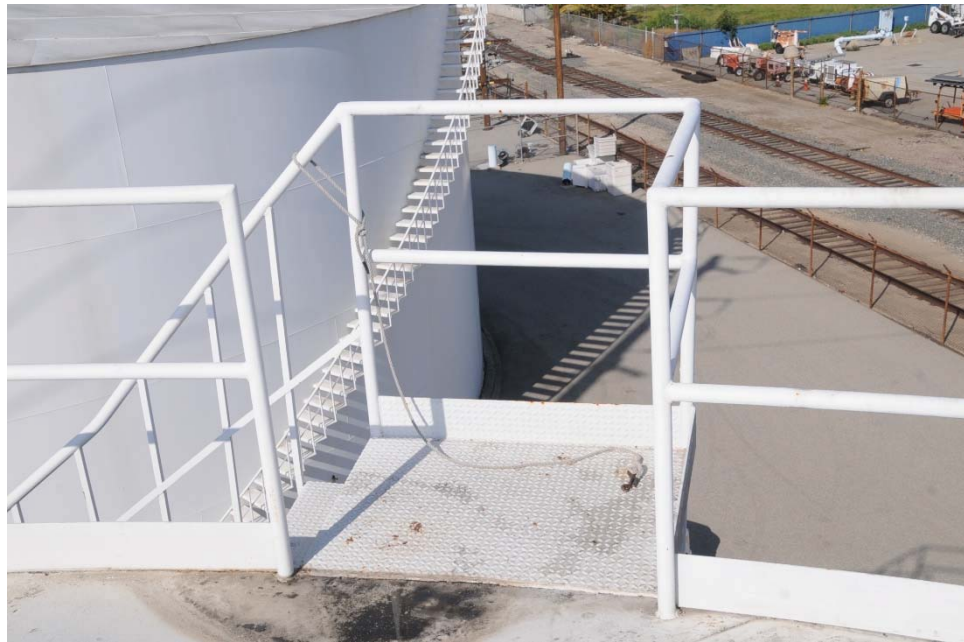
E-15 View of the stairway platform, illustrating random minor spots of corrosion on the platform and guardrailing.
