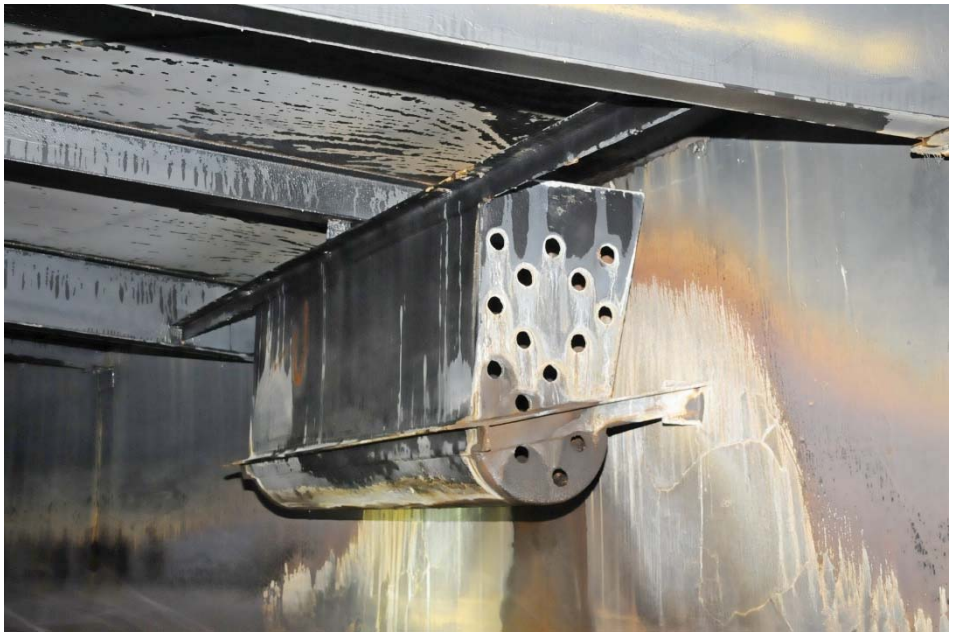
I-26 View of the inlet weir box, illustrating staining on the weir box and adjacent shell.
