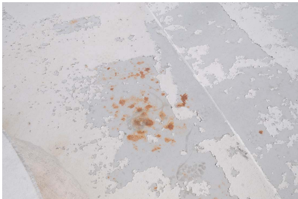
E-10 Same as Photo E-9, except a close-up view of one of the areas of corrosion.
