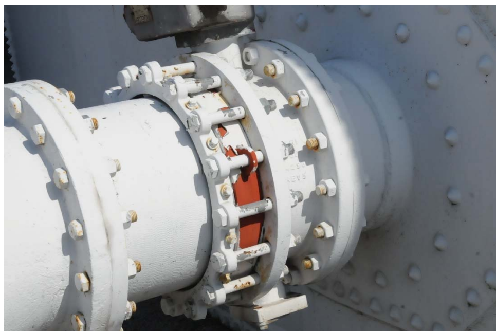
E-31 Same as Photo E-30, except a close-up view of the delamination and exposed prime coat.
