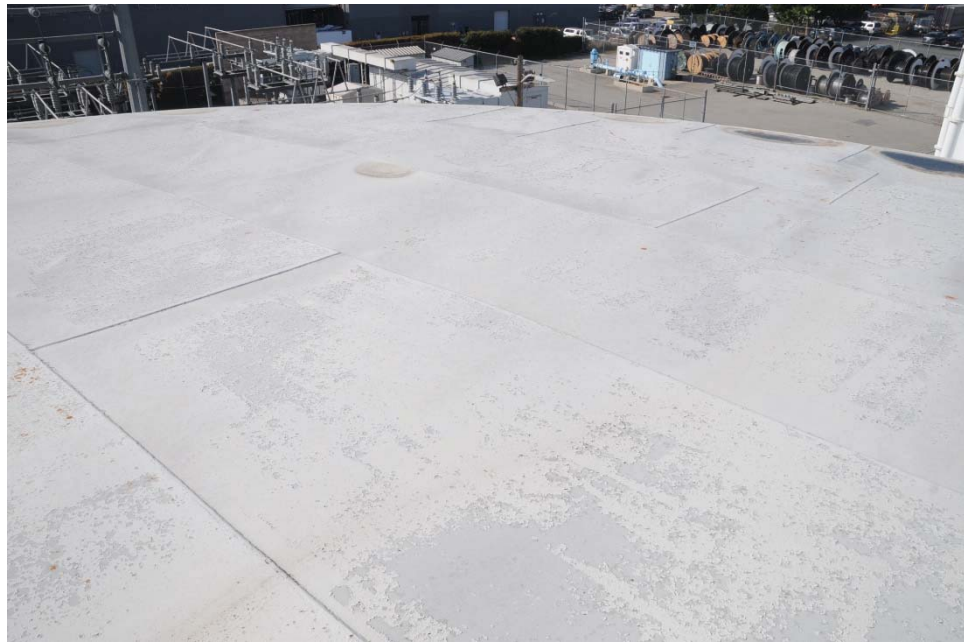
E-8 View of a portion of the roof, illustrating severe delamination of the topcoats.
