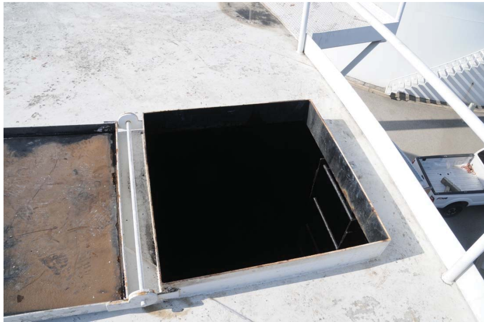
E-14 View of the roof hatch, illustrating minor corrosion at the edge of the hatch curb.
