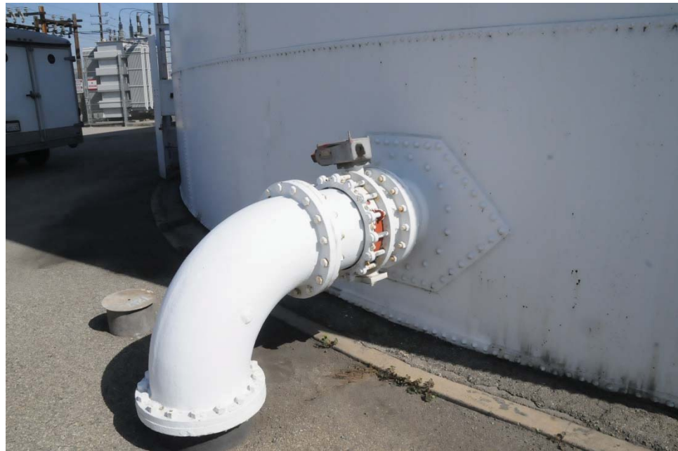
E-30 View of an inlet/outlet, illustrating random corrosion on the nuts and bolts and exposed prime coat on the compression flange.
