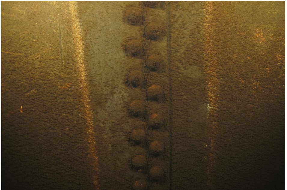
I-45 Same as Photos I-43 and I-44, except in a different location. Note streaks of coating can be seen through the heavy residue in this location.
