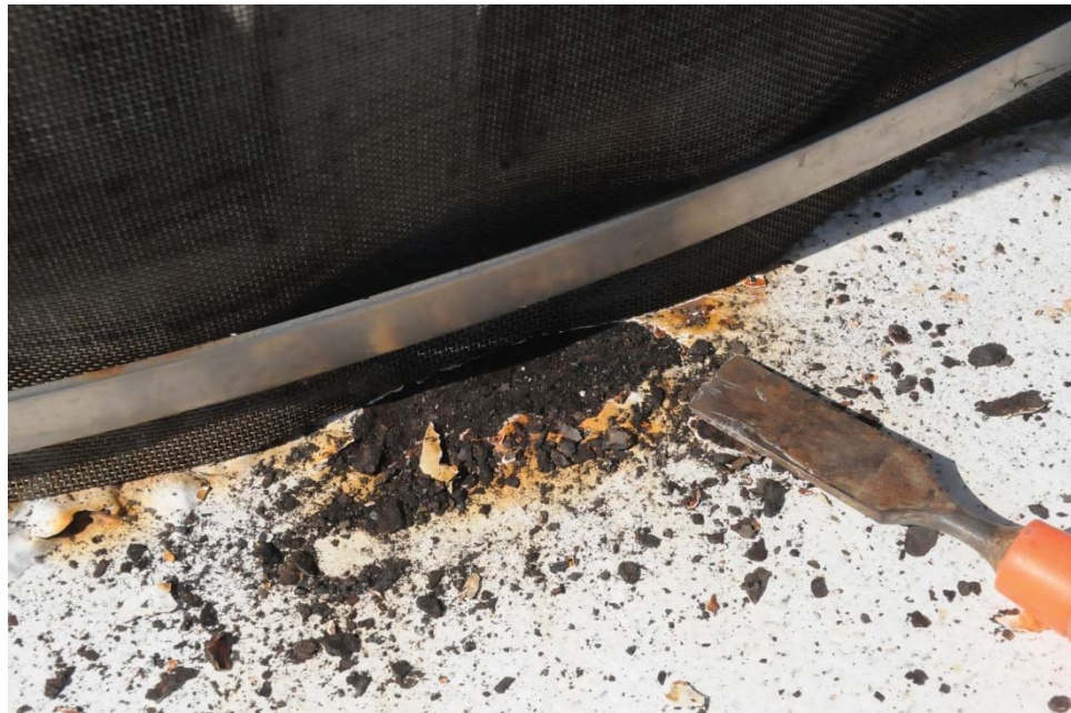
E-6 Same as Photo E-5, except after the rust scale and blister were removed, exposing severe corrosion and a hole in the roof plate.
