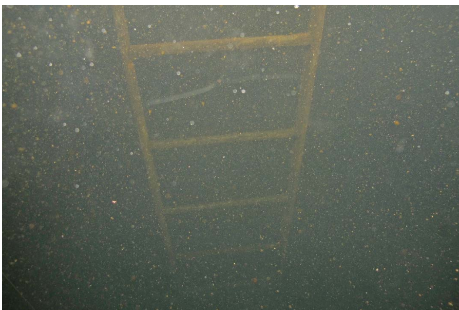
I-33 View of the ladder just below the waterline, illustrating brown staining on the ladder and poor visibility due to contaminants in the water.
