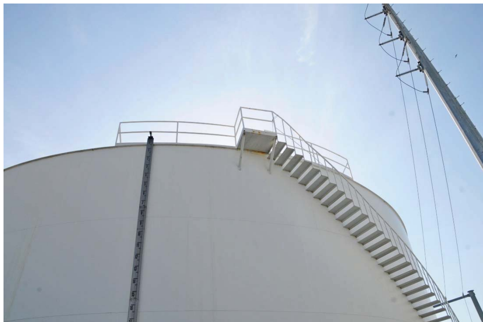
E-19 View of the upper portion of the shell, LLI gauge board, and stairway, illustrating corrosion on the underside of the platform and generally good condition of the shell and LLI gauge board.
