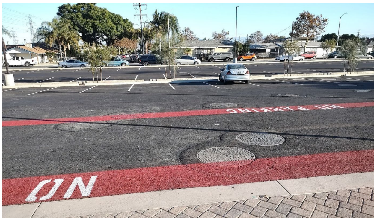
Figure 1-2. John Anson Ford Park Parking Lot Cistern Utility Access Holes.
