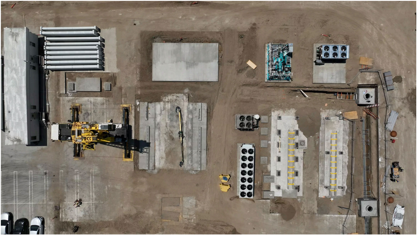
A view of construction at the new Avina Clean Hydrogen Facility in Vernon. It will use large electrolyzer machines powered by 100% clean energy to split hydrogen from water. (Allen J. Schaben / Los Angeles Times)
